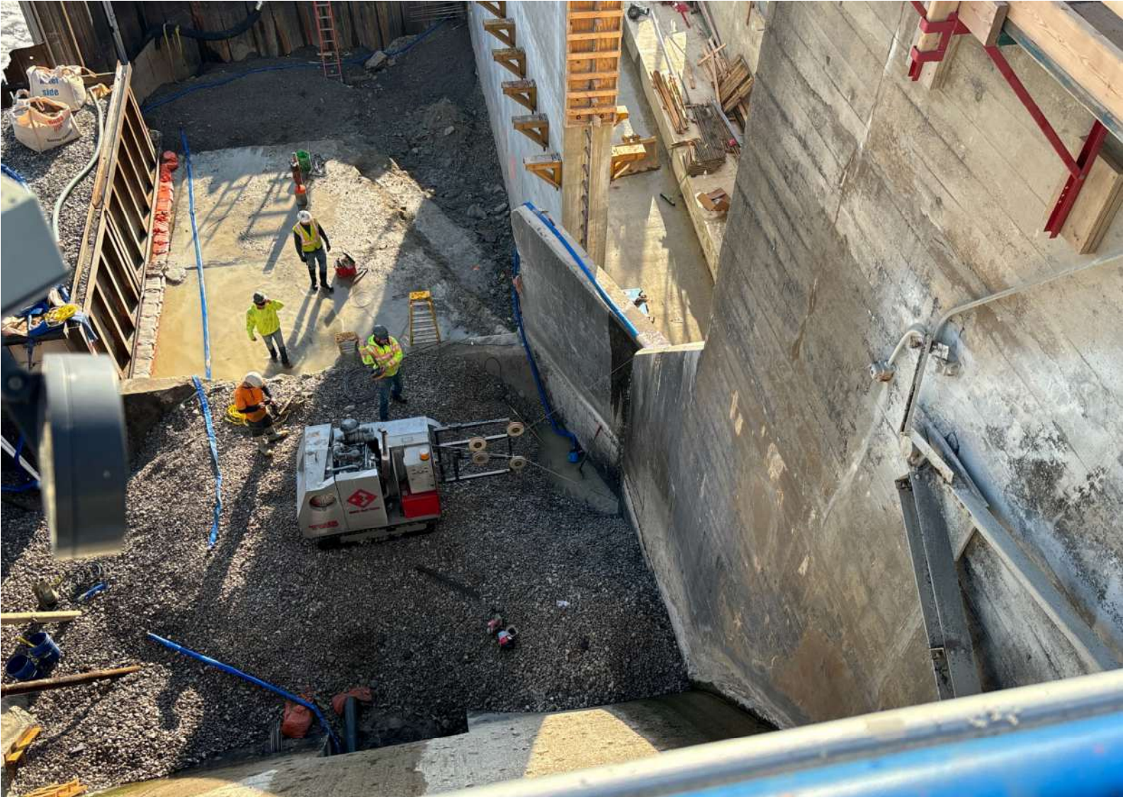
Smallwood Dam – Saw Cutting Existing Right Training Wall
