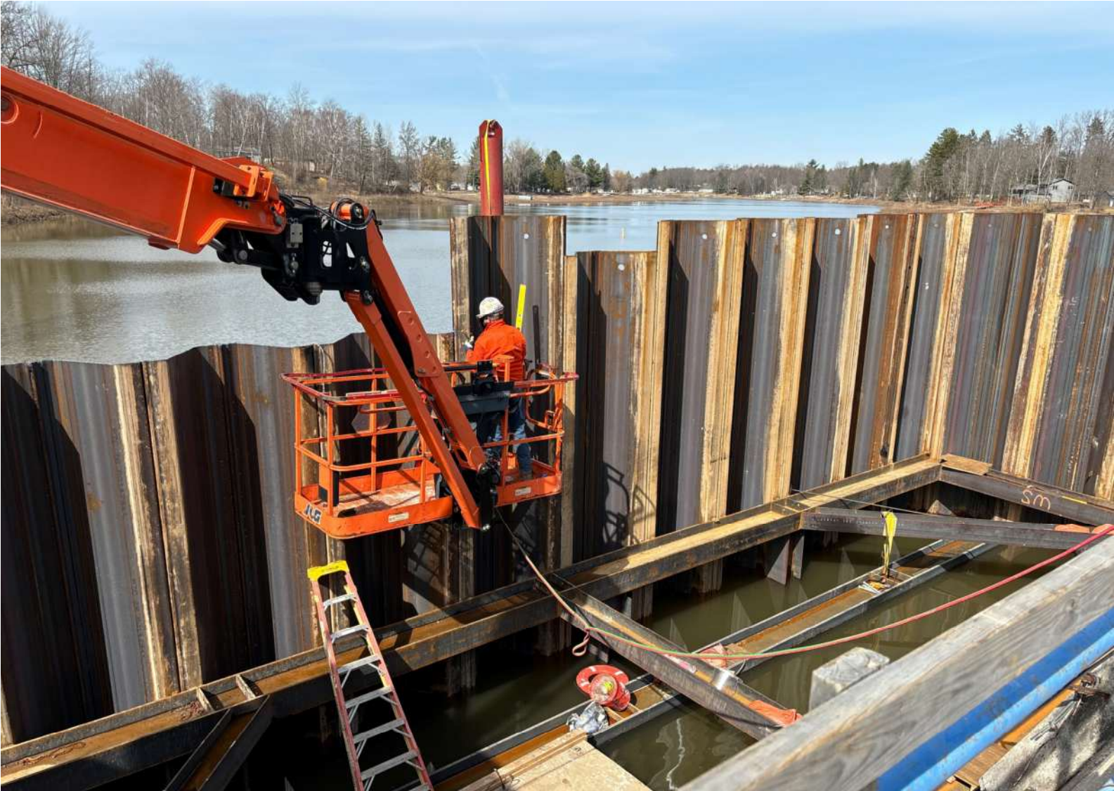
Smallwood Dam – Torching SSP on Upstream Cofferdam to design elevation
