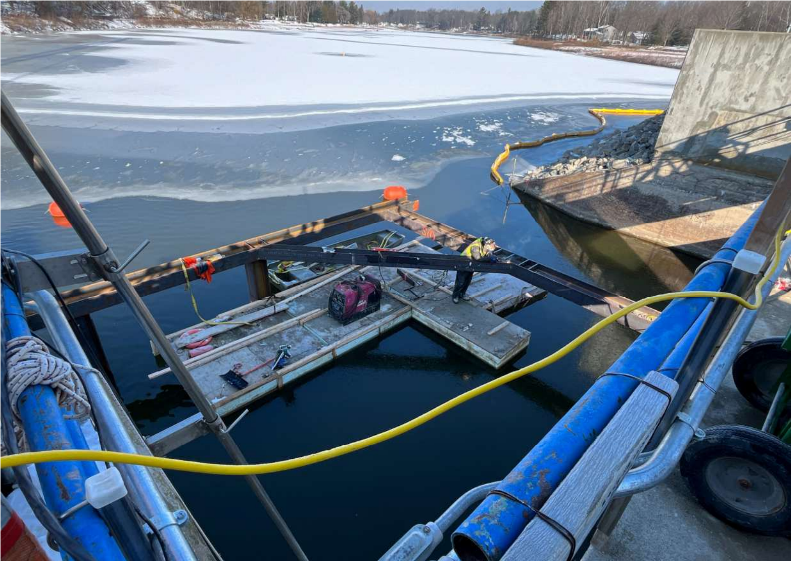
Smallwood Dam – Phase II Upstream Cofferdam Installation
