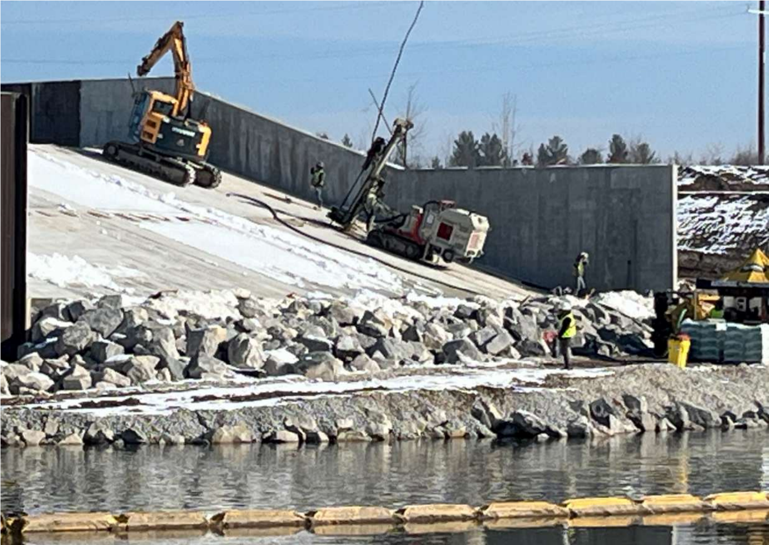
Smallwood Dam – Lower Chute Soil Anchor Installation
