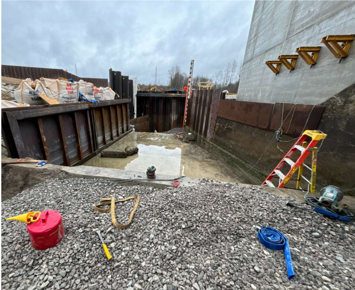
Smallwood Dam – Phase II Downstream Cofferdam Installation
