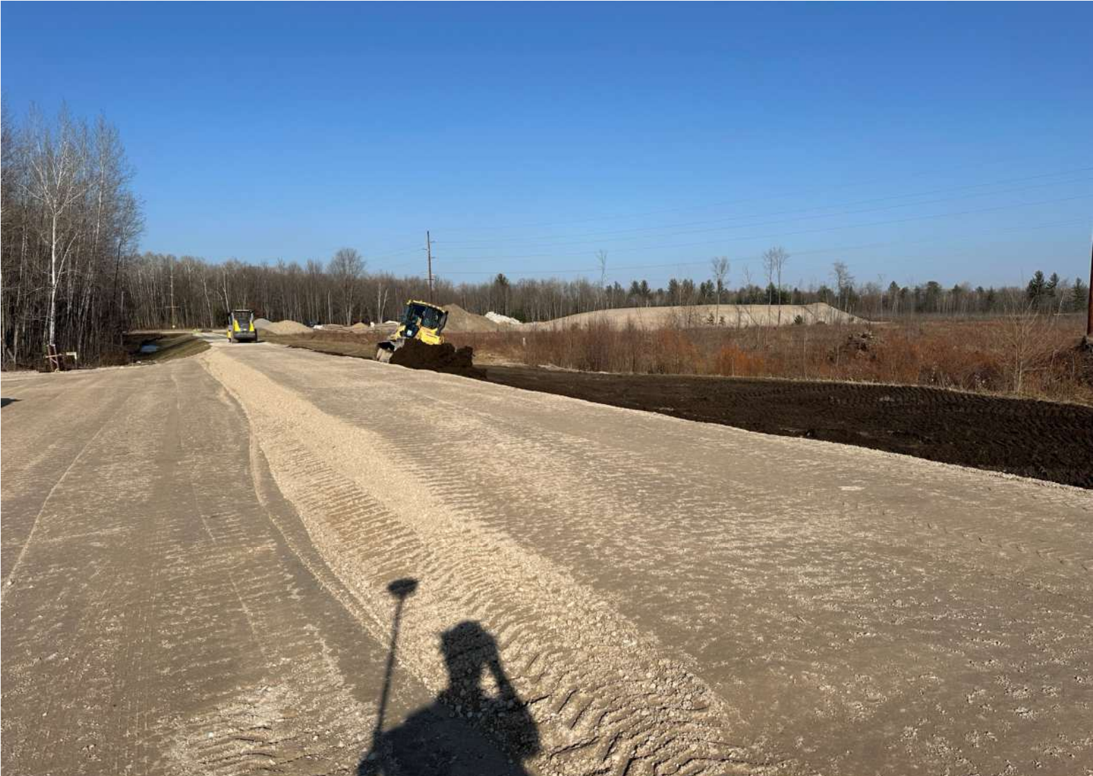
Smallwood Dam – Left Embankment, Placement of Topsoil
