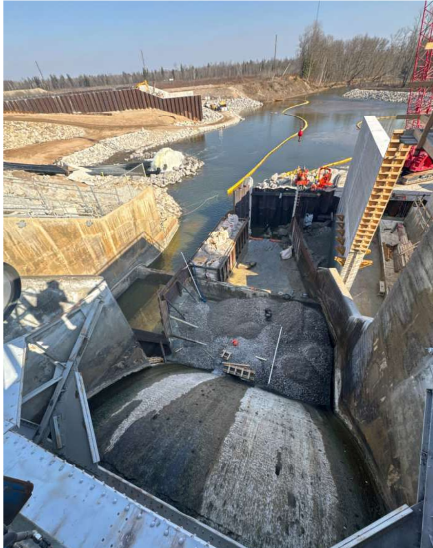
Smallwood Dam – Phase II Downstream Cofferdam Installation
