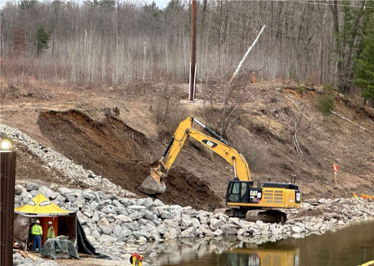
Smallwood Dam – Left Embankment, Stripping Topsoil
