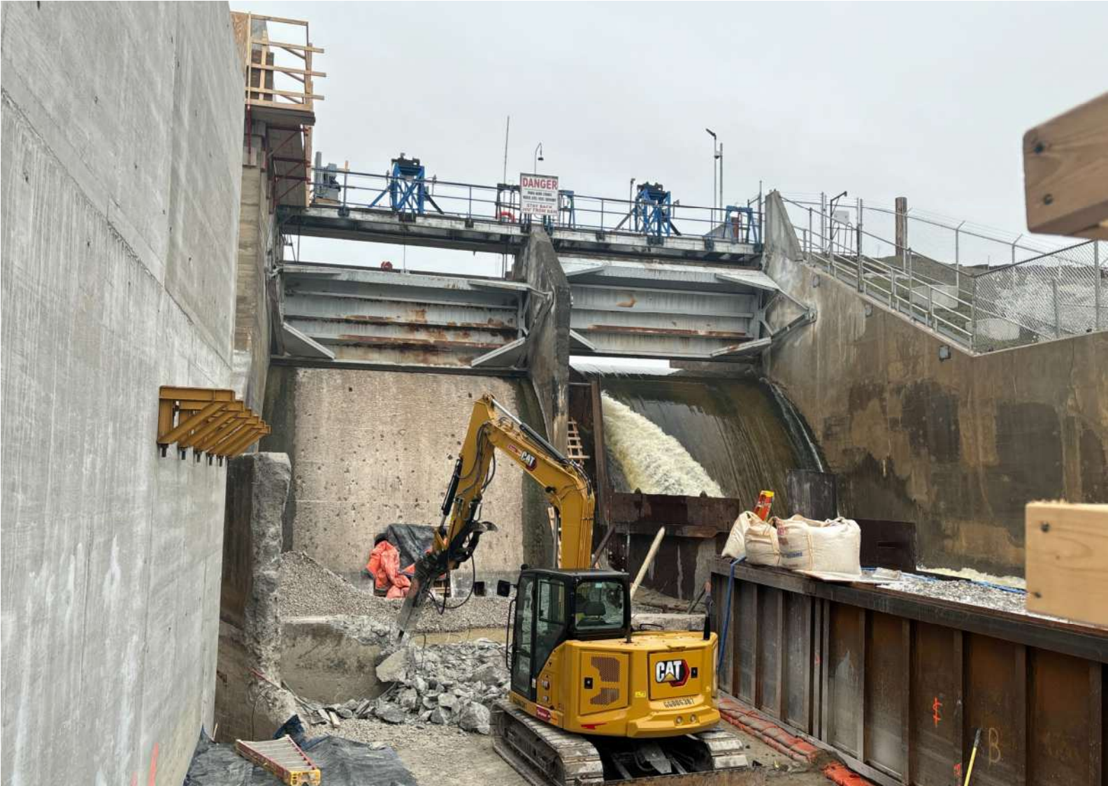
Smallwood Dam – Existing weir demo in primary spillway
