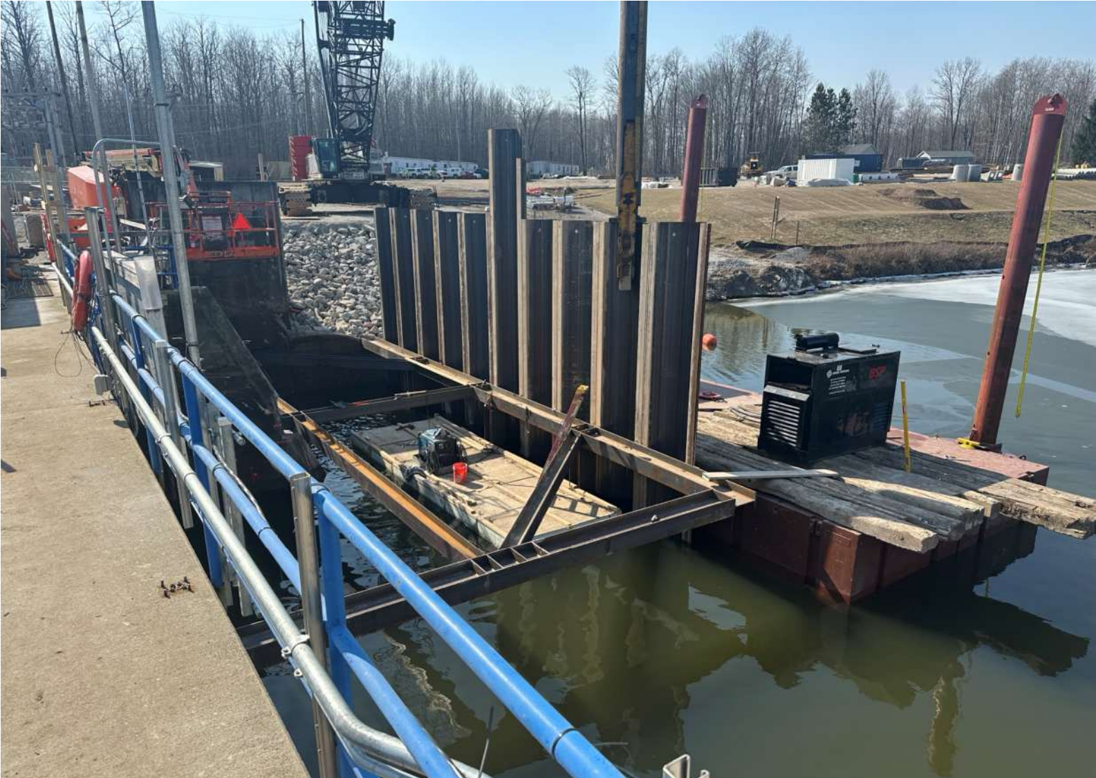
Smallwood Dam – Phase II Upstream Cofferdam Installation
