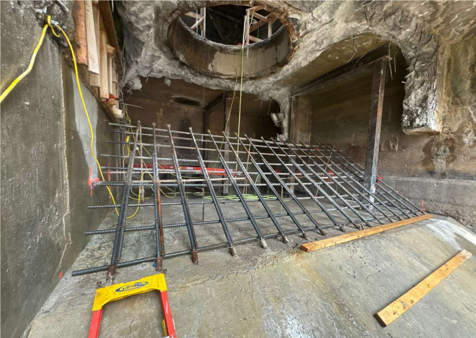
Smallwood Dam – LLO Ramp area
